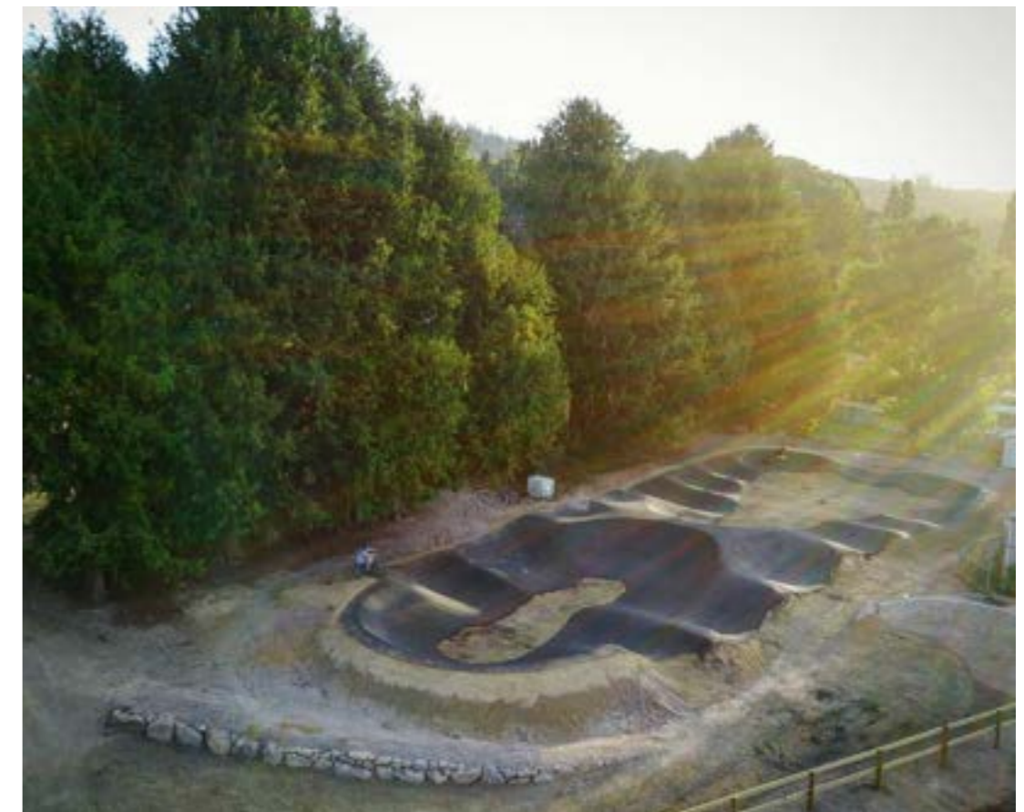
Asphalt pump track
