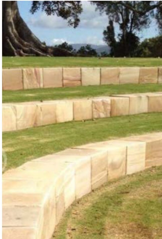
Sandstone retaining and seating walls
