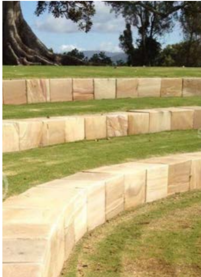
Sandstone retaining and seating walls
